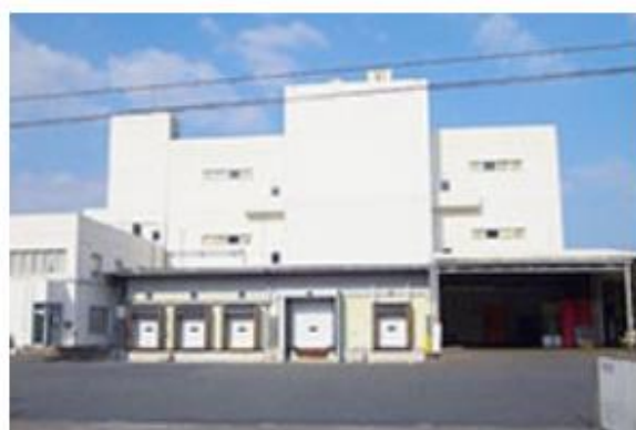
Exterior view of Karatsu Logistics Center
