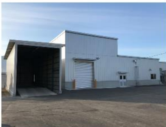
Mechanical building where the biogas power generator is installed
