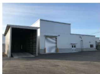
Mechanical building where the biogas power generator is installed
