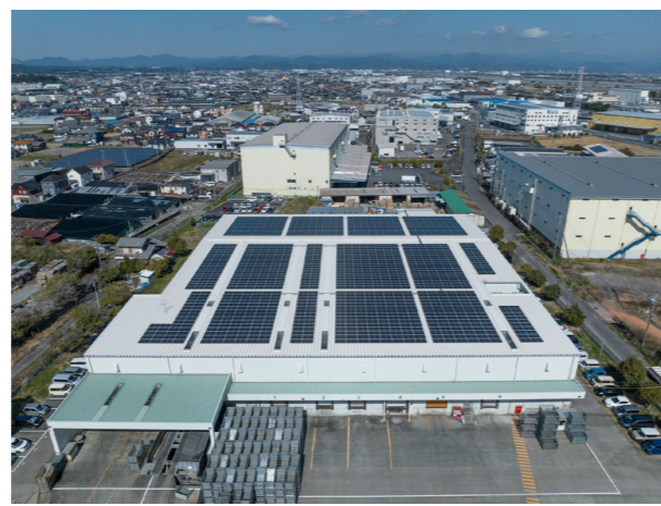
Solar panels installed at Marine Access Corporation (installed in Jan. 2023, estimated to generate approx. 650,000 kWh annually and reduce CO 2 emissions by approx. 260 tons)
